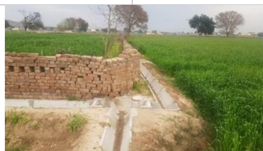
Figure 4.9: Tarnal watercourse branches
