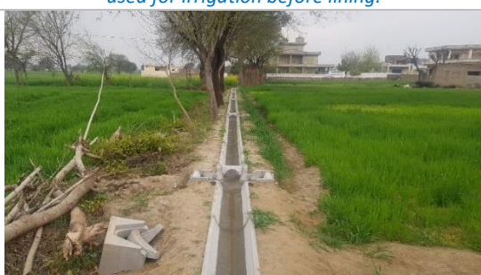
Figure 4.6: Balyala: Lined Watercourse
