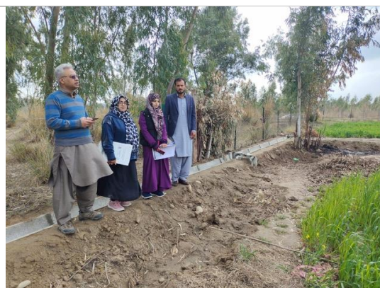
Figure 4.12: Newly Constructed Watercourse
