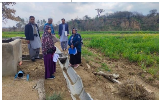
Figure 4.13: Sokason Watercourse Under Construction
