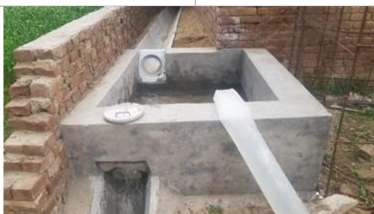
Figure 4.5: Balyala: Plastic foldable pipes were being used for irrigation before lining.
